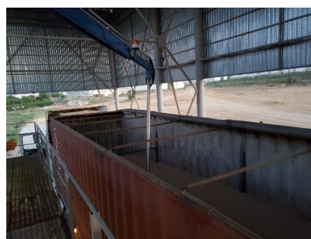
Weighbridge Operations at Nova Dolyna
